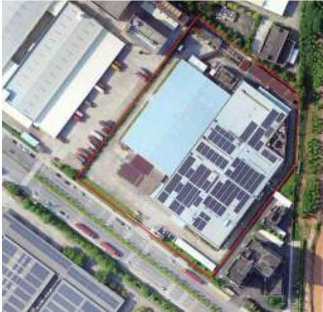
Solar photovoltaic panels in China plant
