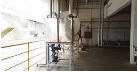
Condensate Recovery System in Cambodia Plant
